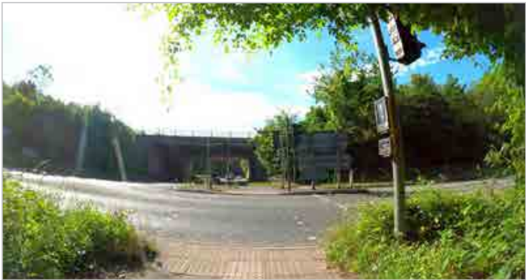
240.1.6 – Hockley Link pavement and crossings
