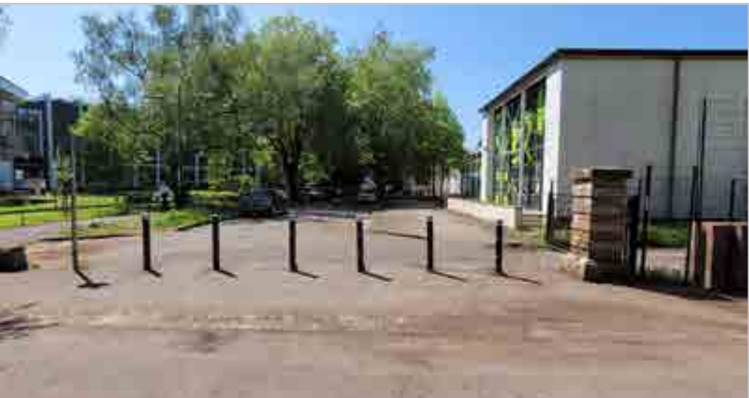
290.2.8 – Park Avenue bollards
