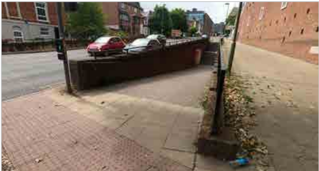
CZ1.1.12 – Access to subway on Sussex Street
