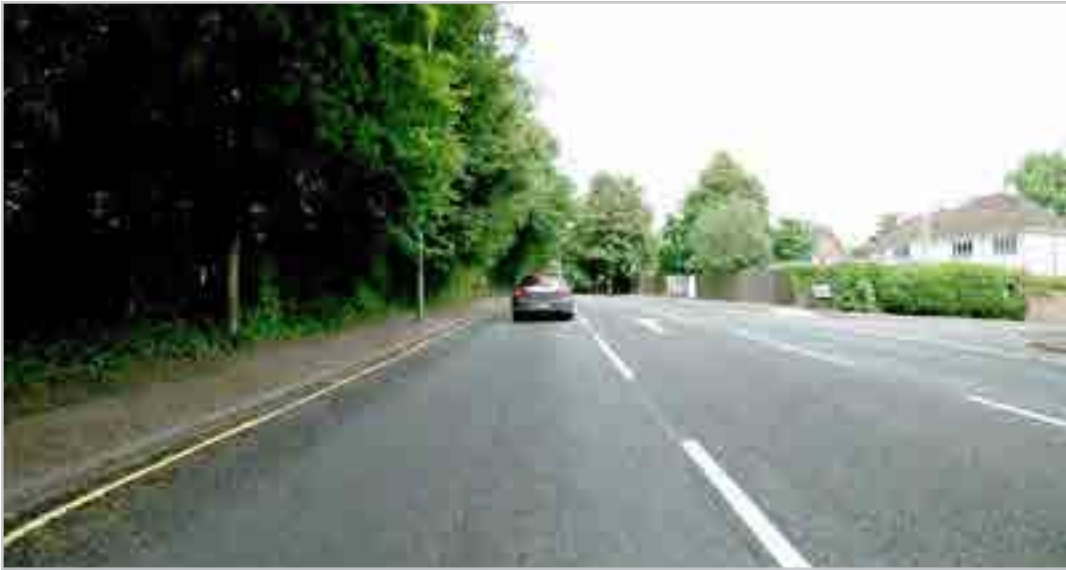
310.1.2a – Chilbolton Avenue and Bath Place
