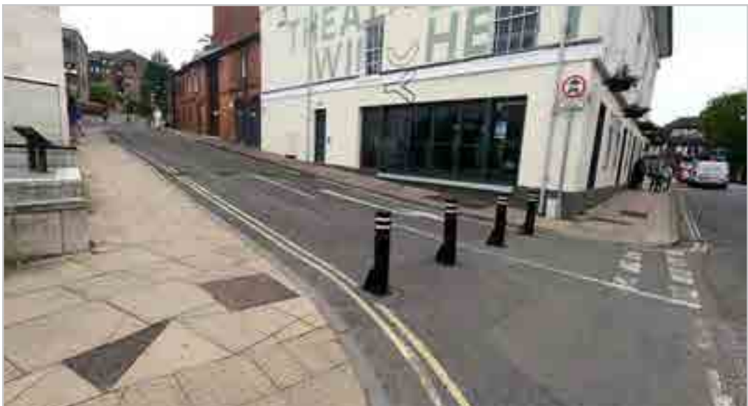
CZ1.2.10 – Jewry Street/Tower Street junction
