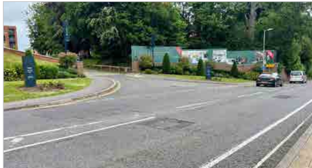
WR8.1.5(c) – Romsey Road/Fellowes Rise junction
