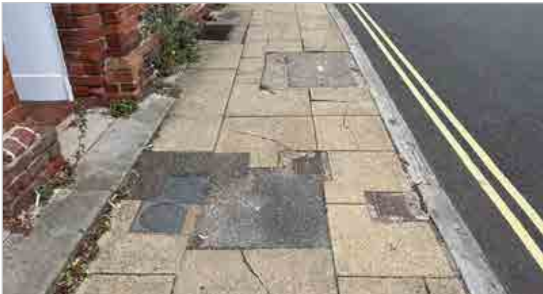
WR3.1.4(c) – Hyde Street pavement
