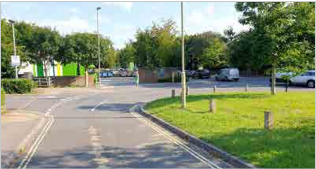
270.1.3 – Burnett Close/Stockbridge Road junction
