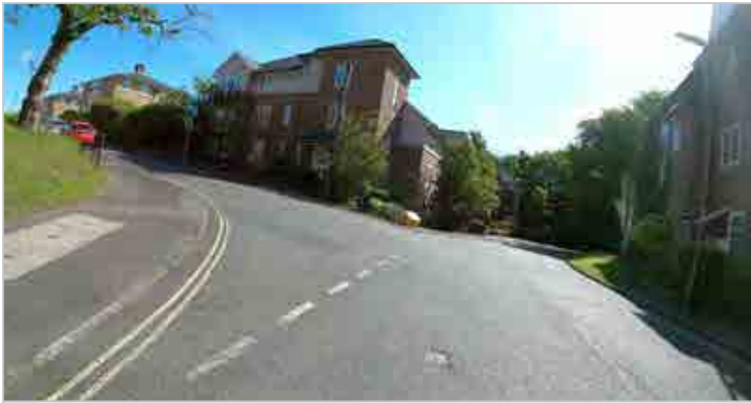
260.2.14 – Greenhill Road junction
