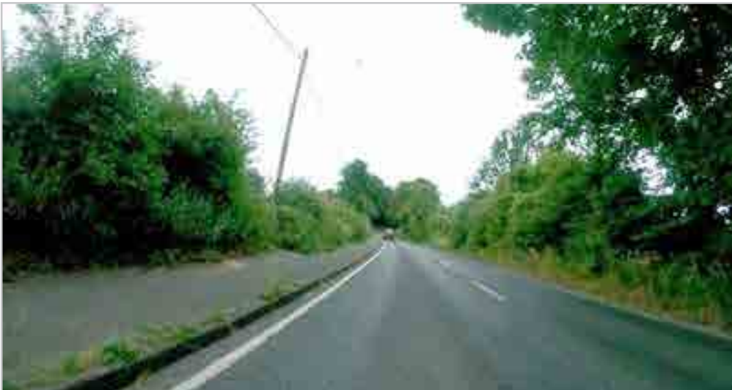
220.1.1 – Worthy Road south of School Lane
