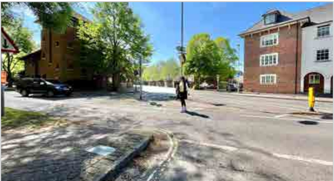
WR5.1.5 – Union Street/North Walls junction
