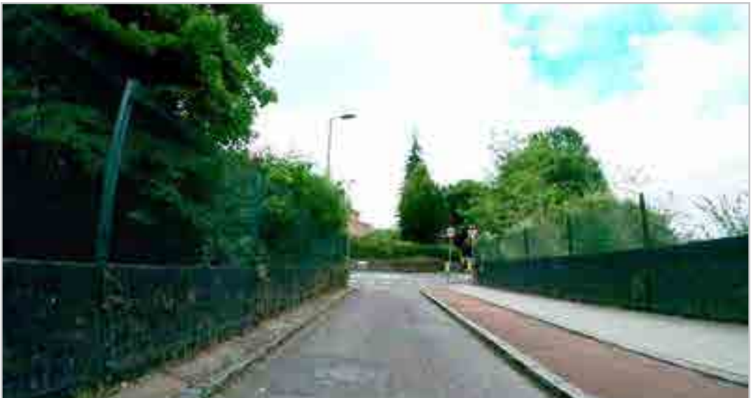
270.2.1 – Upper High Street bridge
