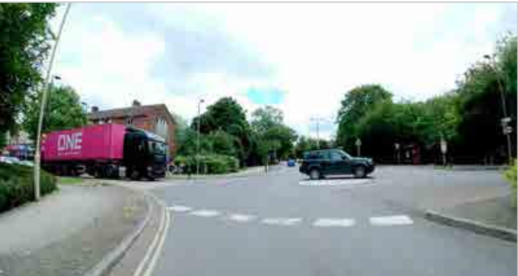
270.1.4 – Stockbridge Road/Stoney Lane junction
