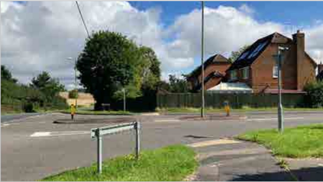
Dropped kerbs w/tactile paving Necessary to create inclusive, accessible crossing points for pedestrians.
