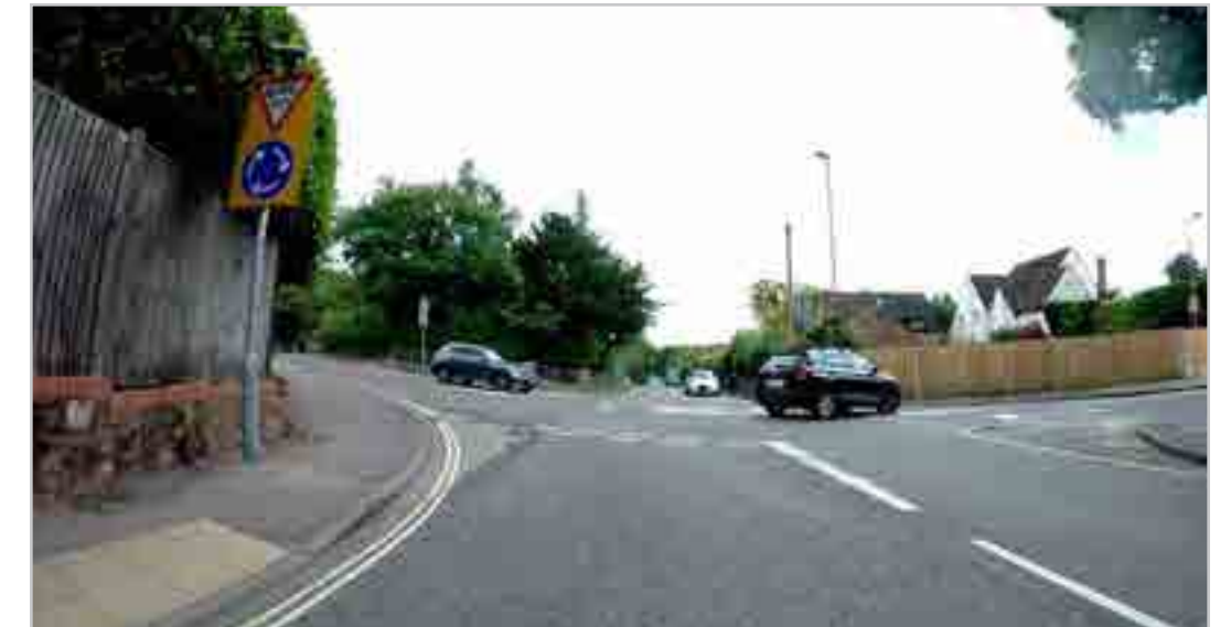
320.1.1 – Stockbridge Road/Bereweeke Road junction
