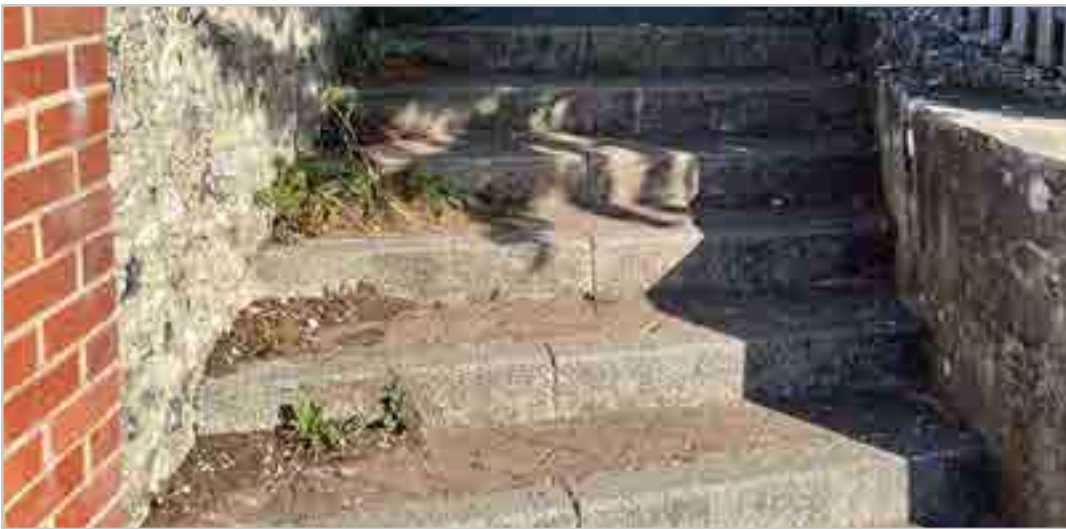
WR2.1.4 – Steps at Cattle Market car park at Worthy Lane
