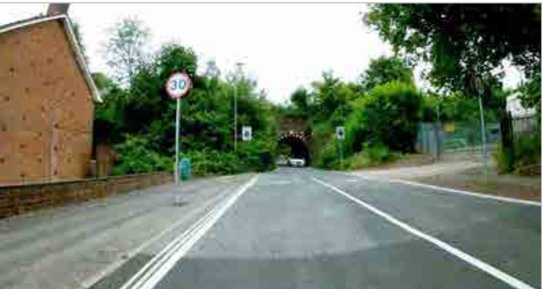
250.1.8 – Lower Stanmore Lane railway underpass
