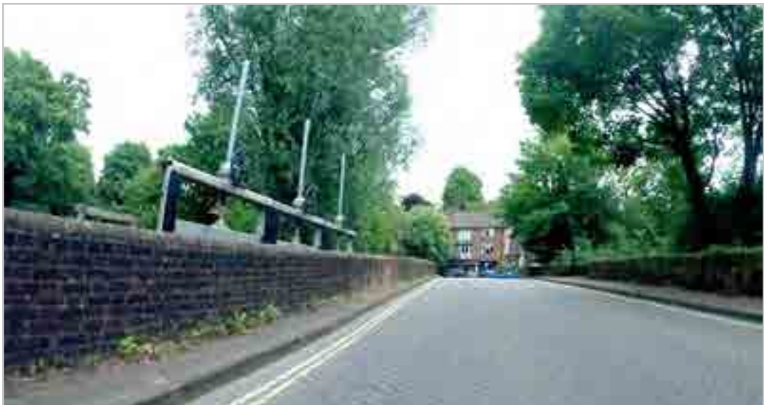
300.1.1 – Durngate Place and Easton Lane
