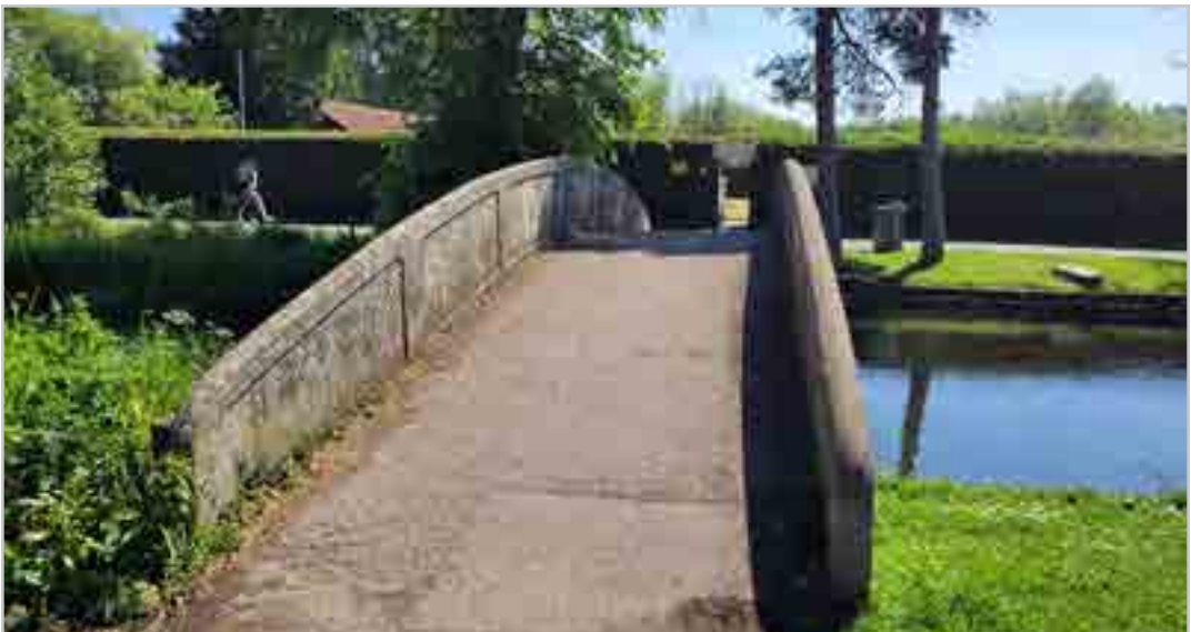
290.2.6 – River Recreation Ground Park bridge
