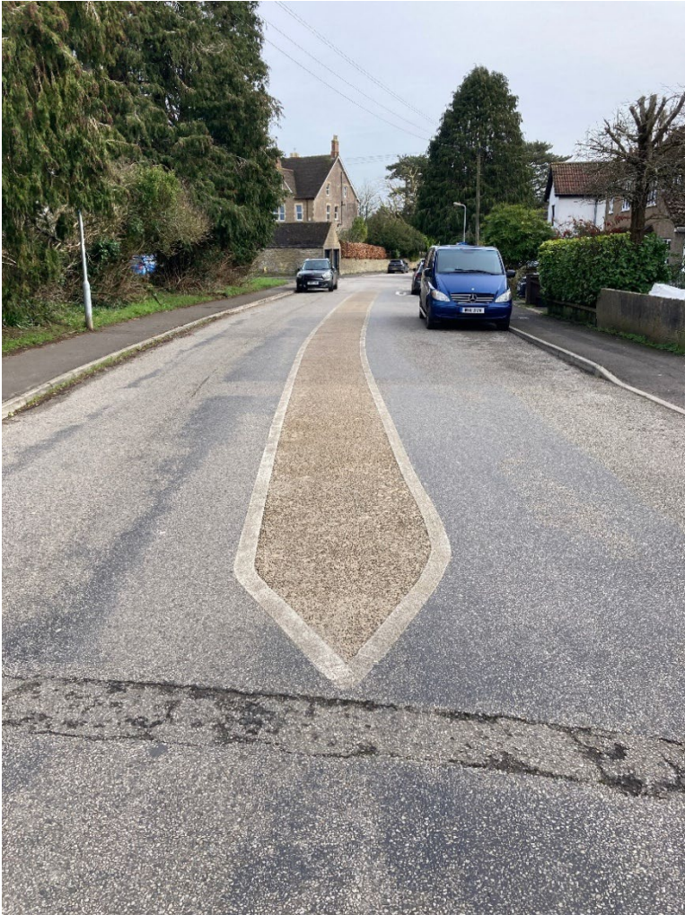
Figure 23 Example of a central median strip
