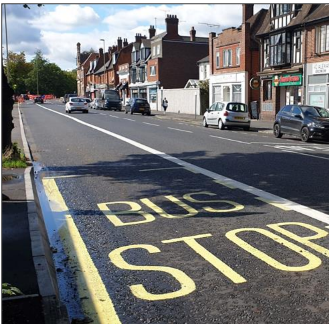
Completion of resurfacing works on Alexandra Road
