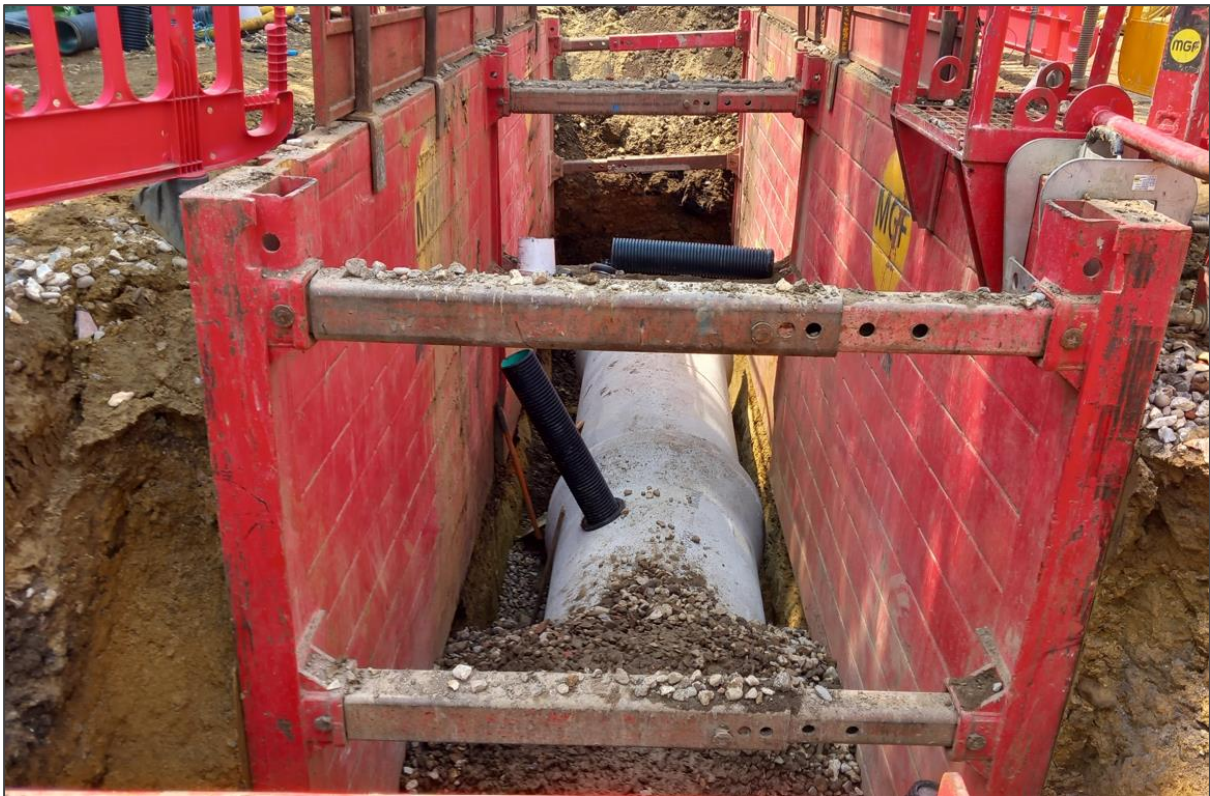
A3011 Lynchford Road - Deep drainage.
