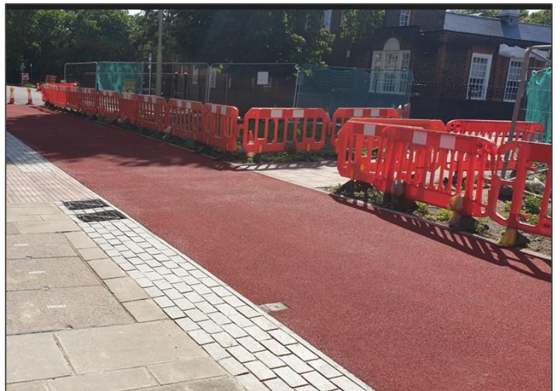
Alexandra Road– Anti skid coloured surfacing for the cycleway
