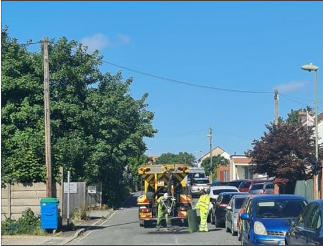
Gordon Road – Surface repair works have now been completed.
