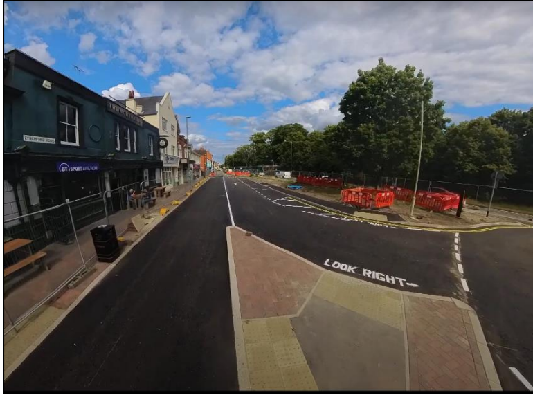
(Old) Lynchford Road – New junction with A3011 Lynchford Road opened
