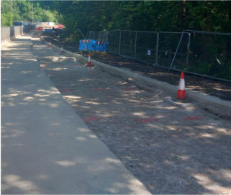
Lynchford Road – Carriageway widening with new kerb being installed.
