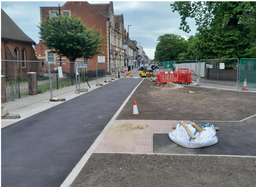
Alexandra Road - by St Alban's roundabout, surfacing, tactile paving and topsoil
