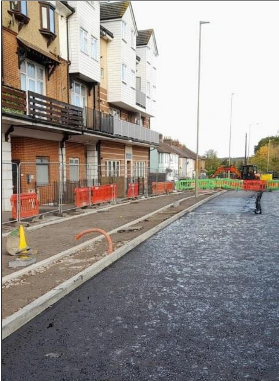
Footway works progressing East of Morris Road
