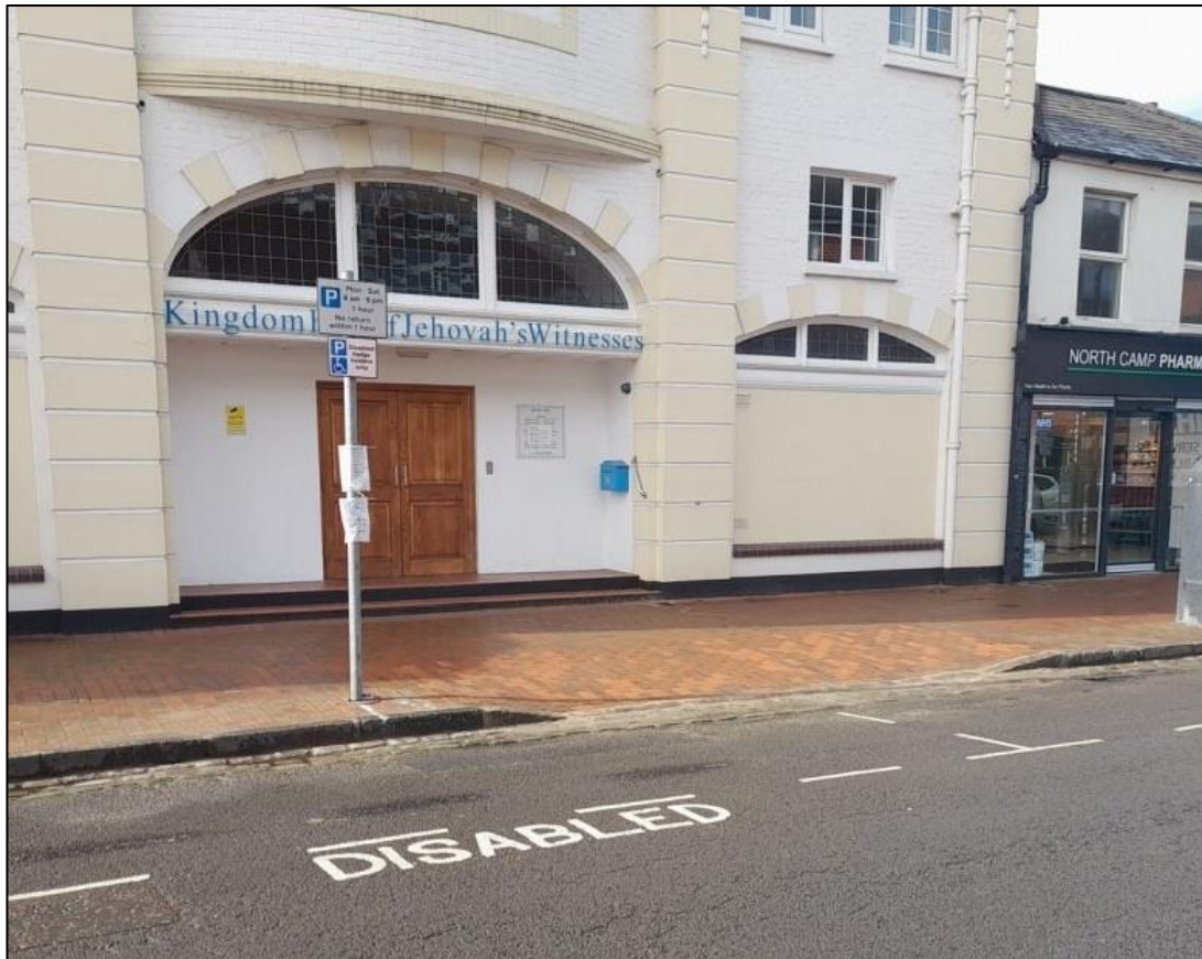
Two new parking bays and dropped kerbs installed along Camp Road
