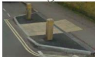
PAVEMENT BUILD OUT
