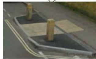
PAVEMENT BUILD OUT
