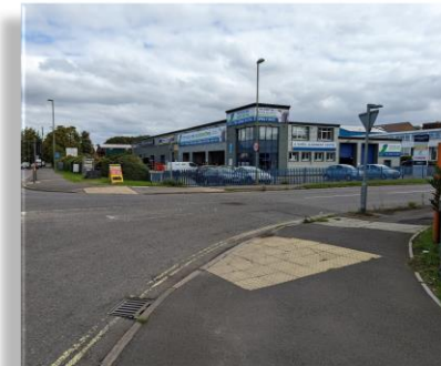
Existing Lister Road junction
