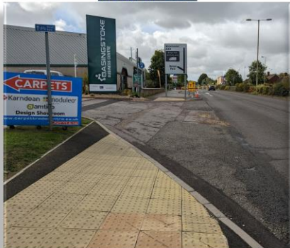
Existing pavement layout along the A30
