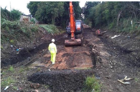
Road excavation and first layering of capping material by Hutfield Link
