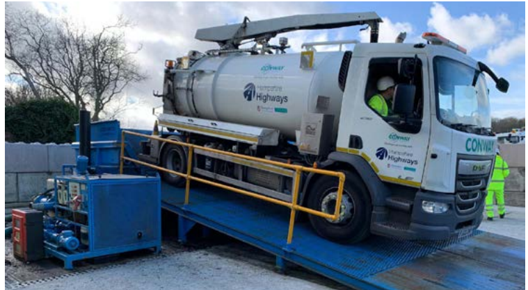
Northington Gully Waste Treatment Plant
