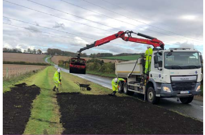
Rewilding trial site in Waterlooille
