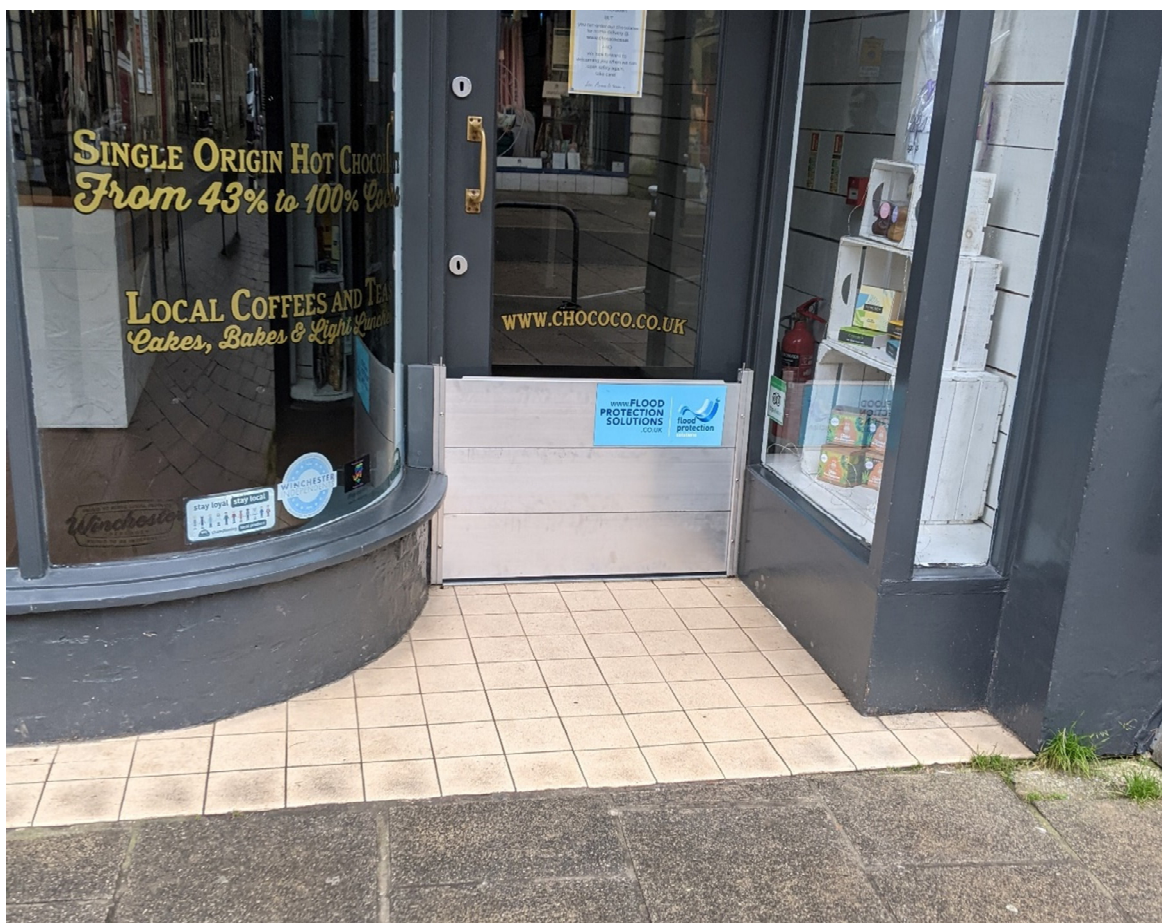
Figure 5-3: Flood barrier installed on property in the High Street
