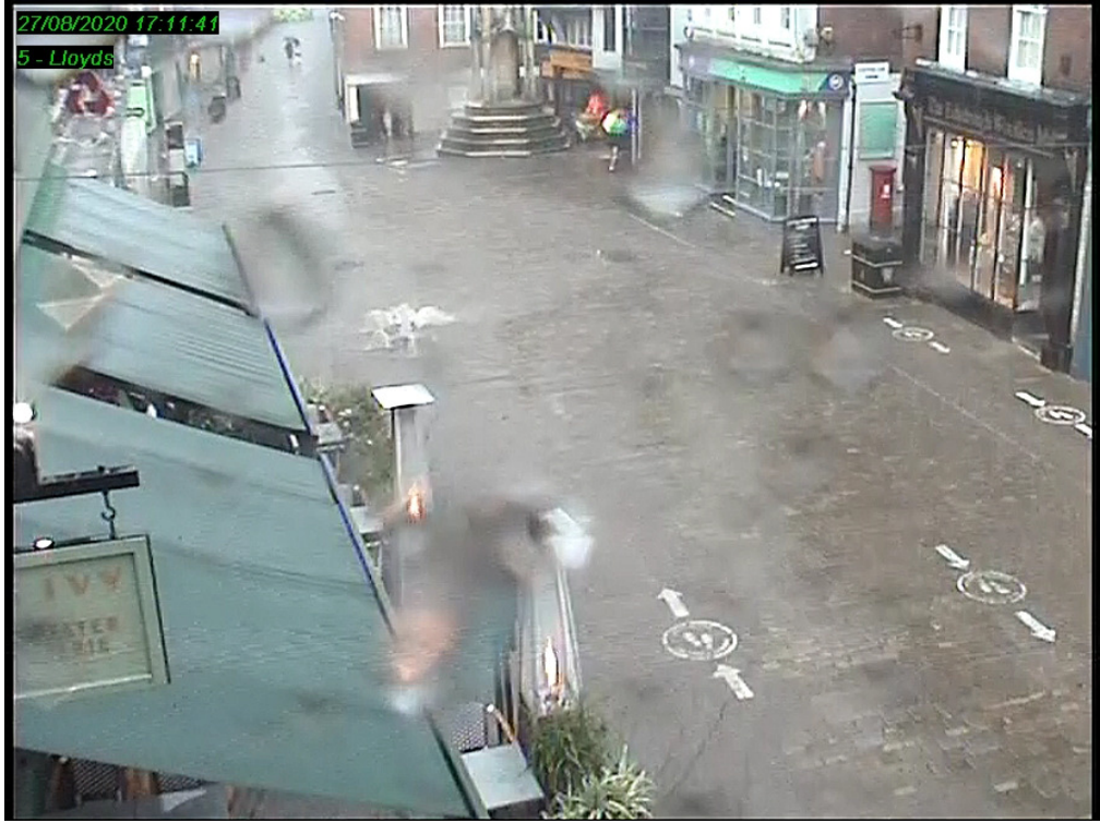
3. Surface water flowing along the High Street (looking east)
