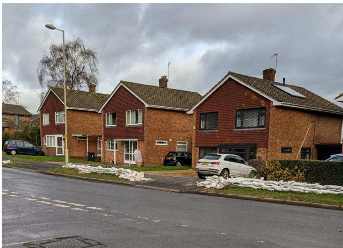
Figure 5-4: Use of sandbags in Harestock
