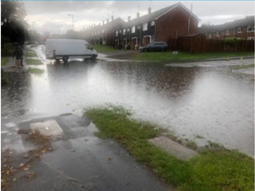
1. Surface water flooding at the junction of Buriton Road and Grayshott Close (looking south)
