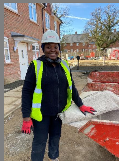
Olu's job involves keeping the site tidy.
