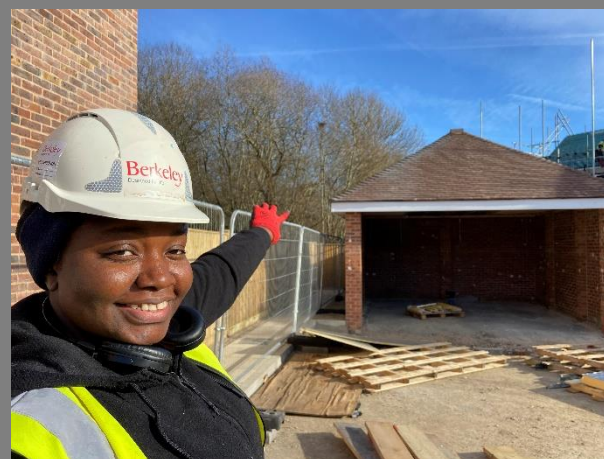
Olu helped tile this roof
