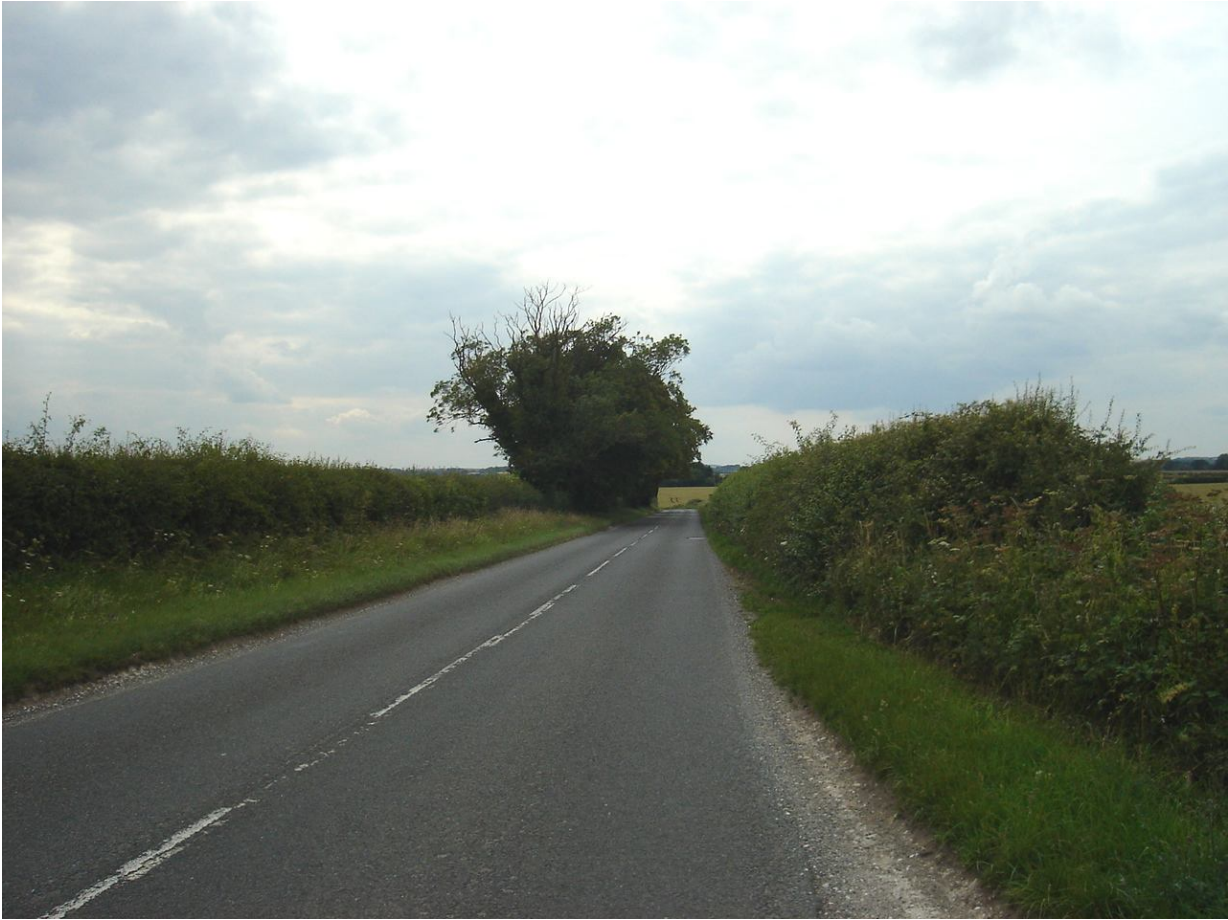
A typical view of Old Stockbridge Road
