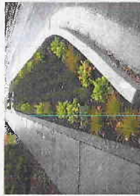
The green built out, forming part of the priority system replaces asphalt with low maintenance planting, helping to slow traffic on approach to the crossing. As well as added safety benefits, the amenity value is also improved.
