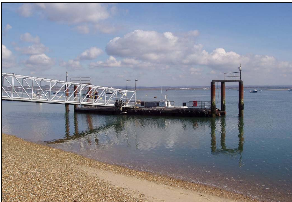
Figure 2.1 – Eastney linkspan, pontoon and dolphins viewed from the south
