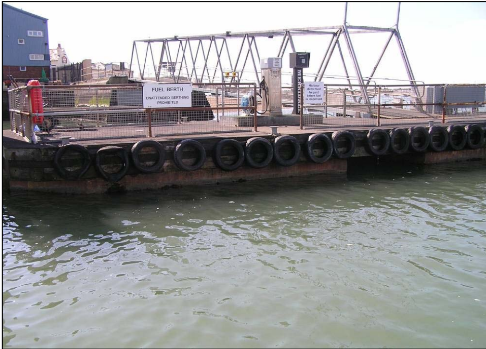
Figure 2.1 – Hayling pontoon and linkspan viewed from the north-east
