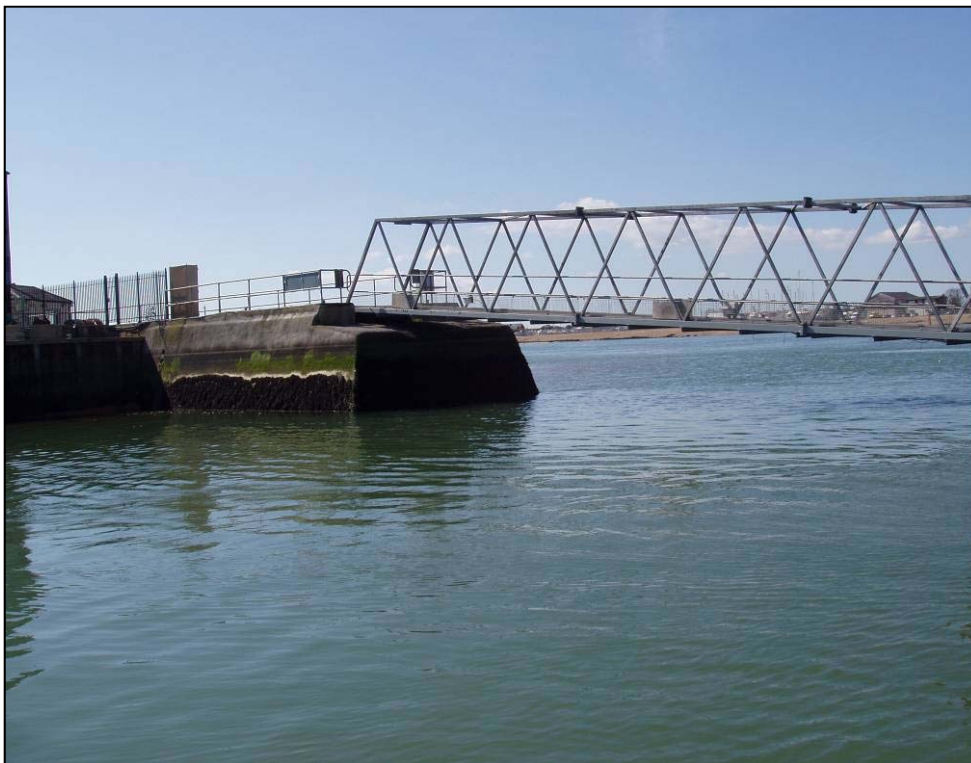
Figure 2.2 Hayling linkspan and fixed approach viewed from the east
