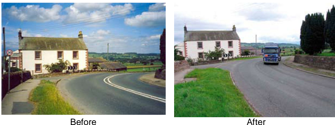
Figure 1: Removal of centre lines in Clifton (DfT, 2008)
