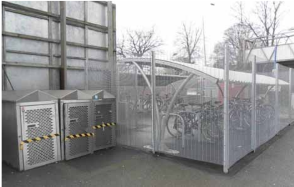
Photo 4.2 - Secure cycle parking at Fleet, as seen from the platform – old cycle lockers to the left are scheduled for removal.
