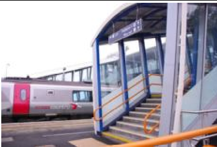
A new accessible footbridge with lifts was completed at Southampton Airport Parkway station in 2009 as shown here (new footbridges were also installed at Fareham and Fratton)
