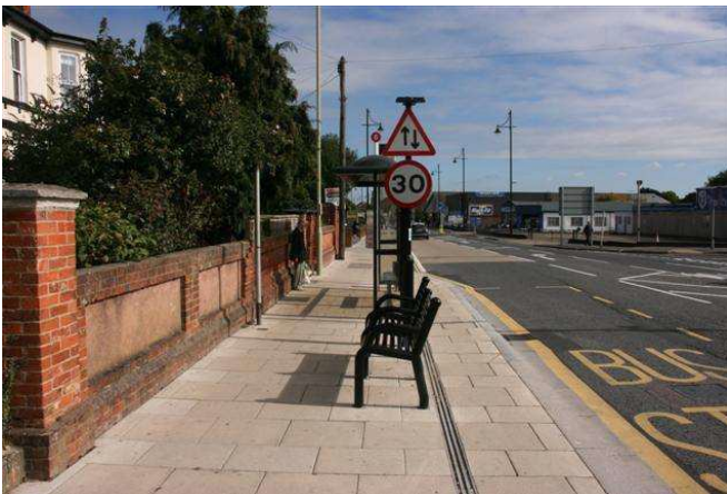
View looking east at the western end of West Street
