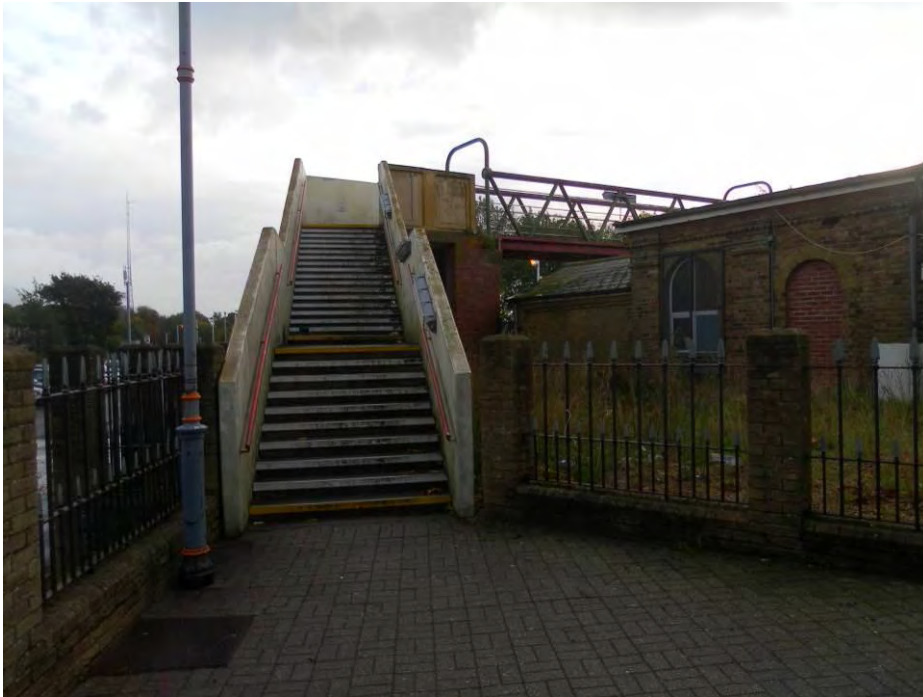
Photo 4.5 - Steps up to the footbridge over the railway from the north side
