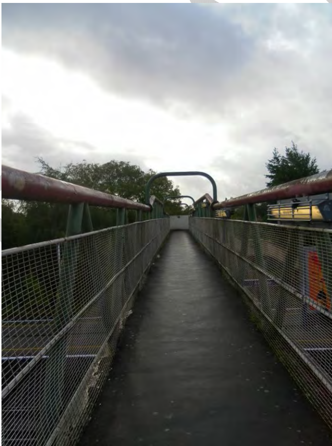
Photo 4.6 - Footbridge over the railway
