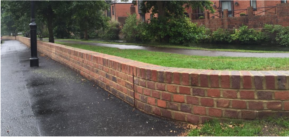
Water Lane Flood Defence Wall
