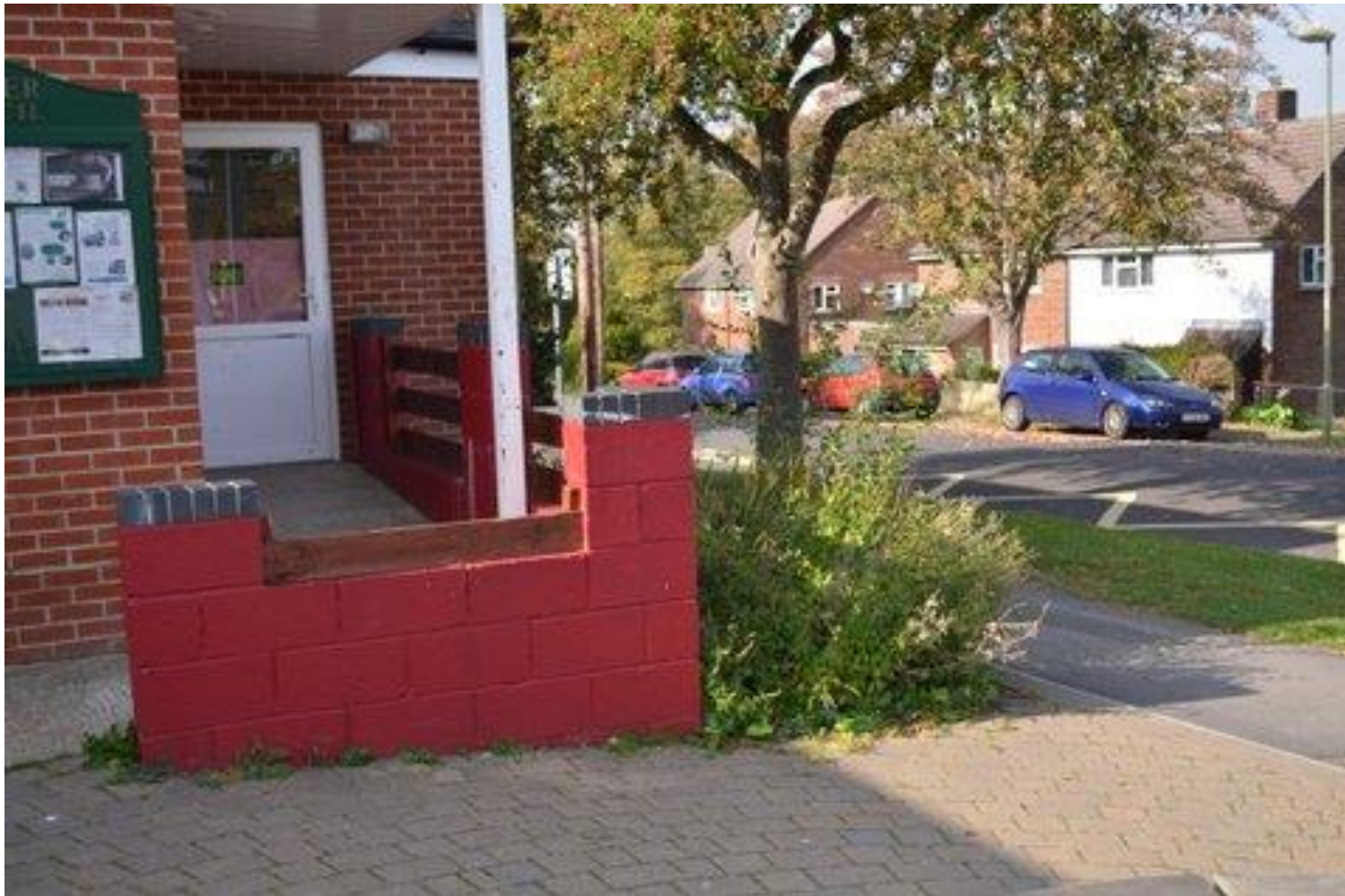
Ramped wheelchair access
