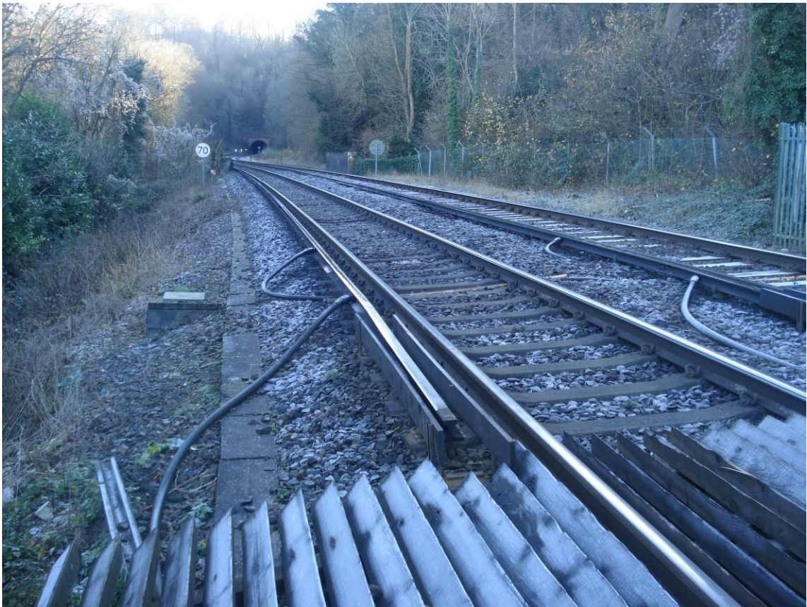
looking SE towards tunnel from recreation ground side
