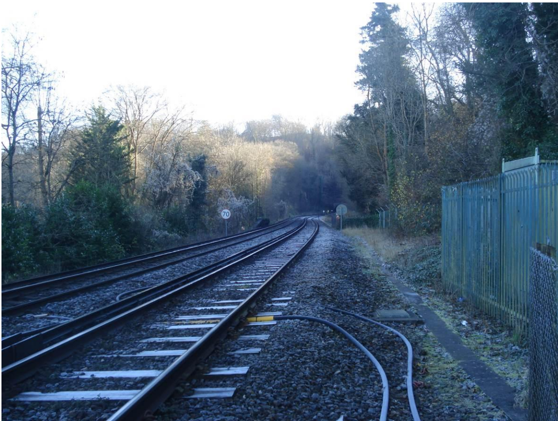
looking SE towards tunnel from Chalk Pit side
