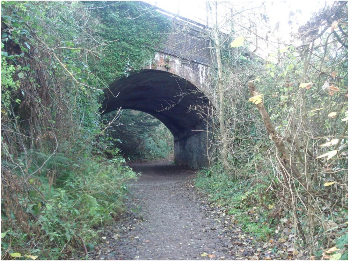
Bridleway 4 at underpass
