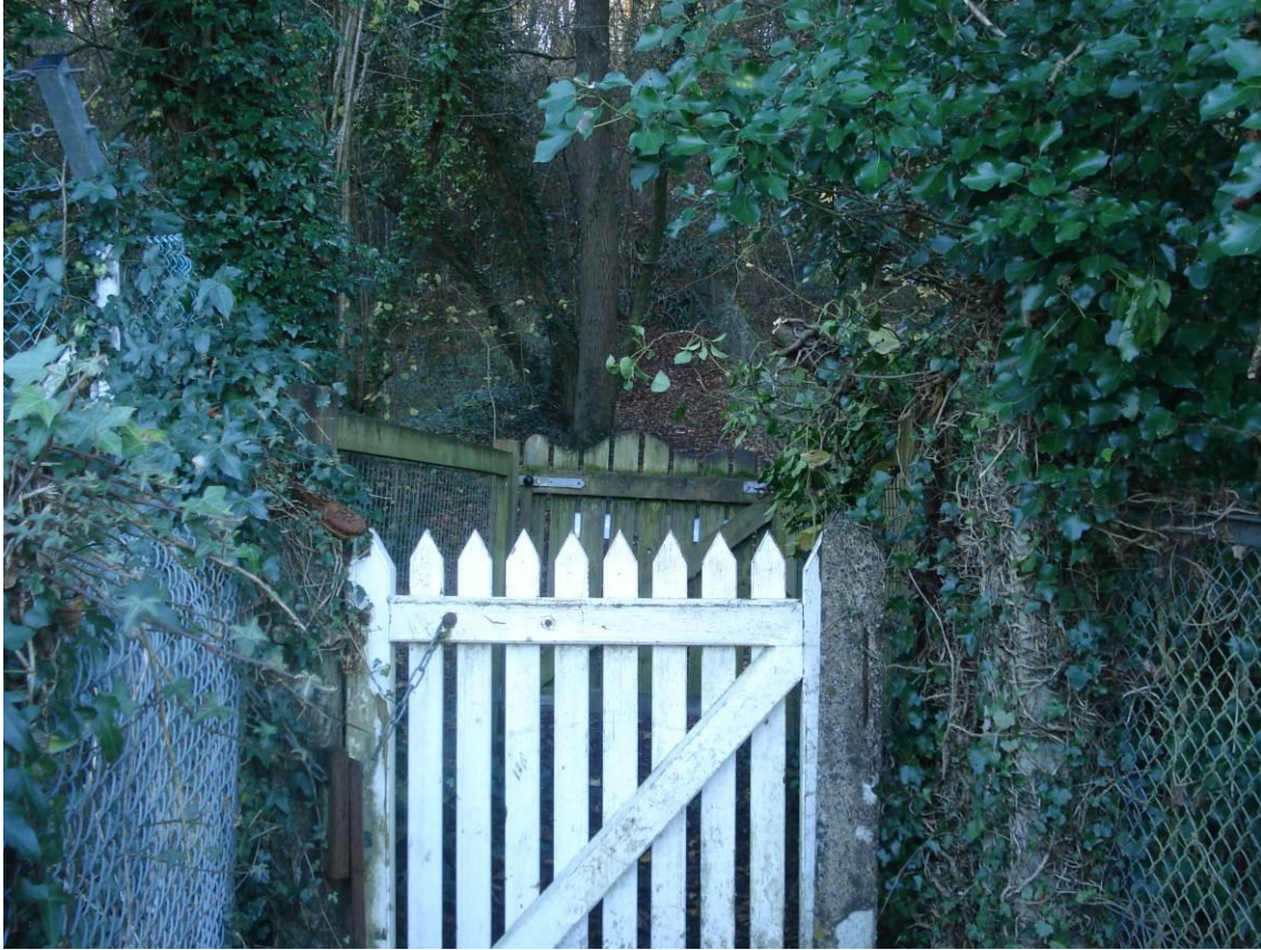
double pedestrian gates on Chalk Pit side
