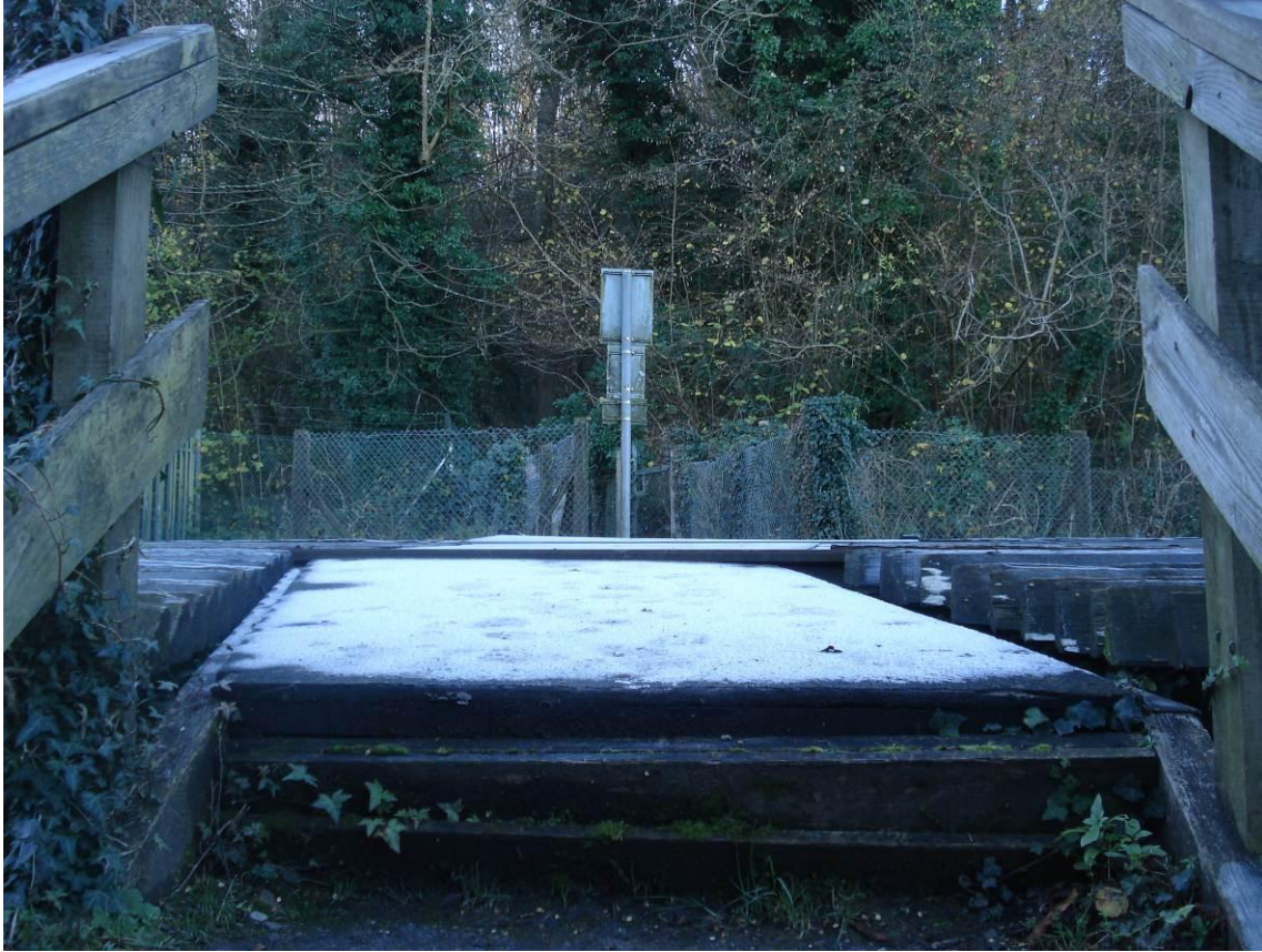
top of steps at crossing deck on recreation ground side
