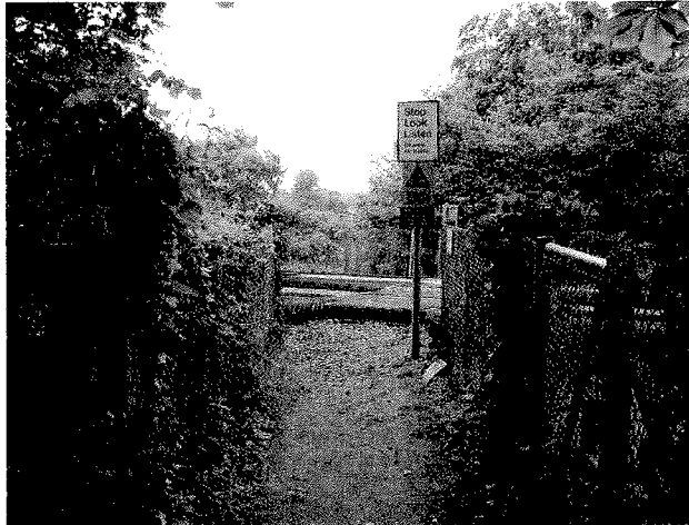
Up side crossing approach
