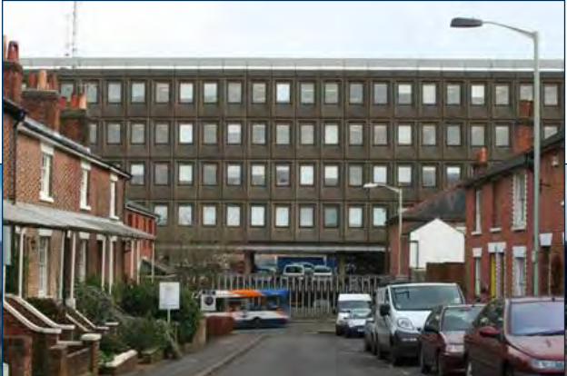
External Facade - before
