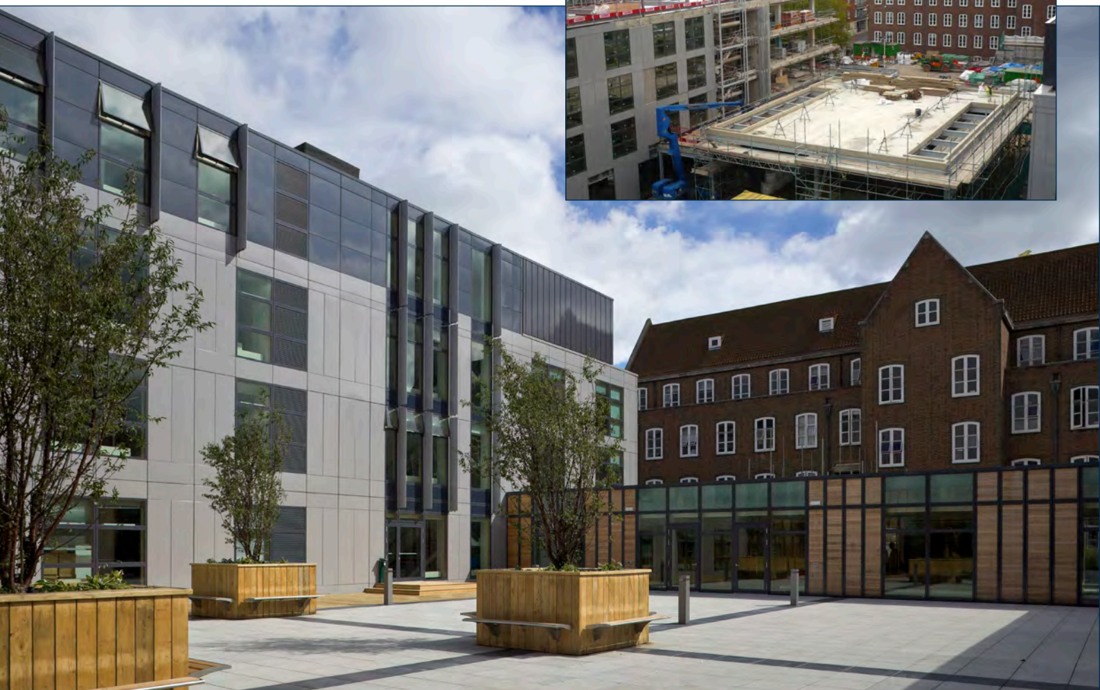
The Courtyard - Elizabeth II Court - after
