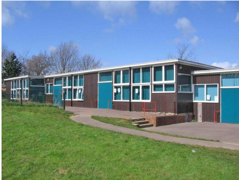
Barncroft Primary School, Hampshire (Before)
