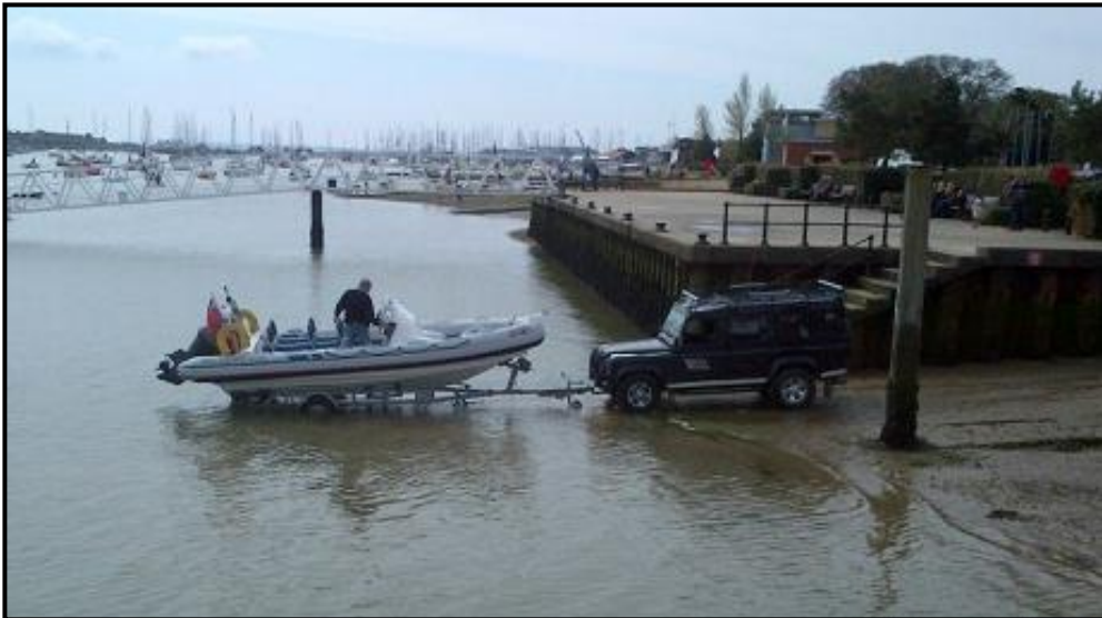
Figure 2.3 Shallow Slipway Gradient Making Vehicular Launch and Recovery Difficult
