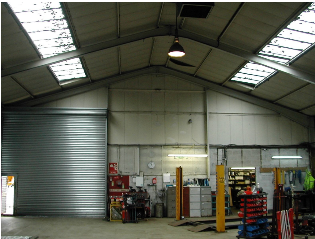
Internal view of workshop
