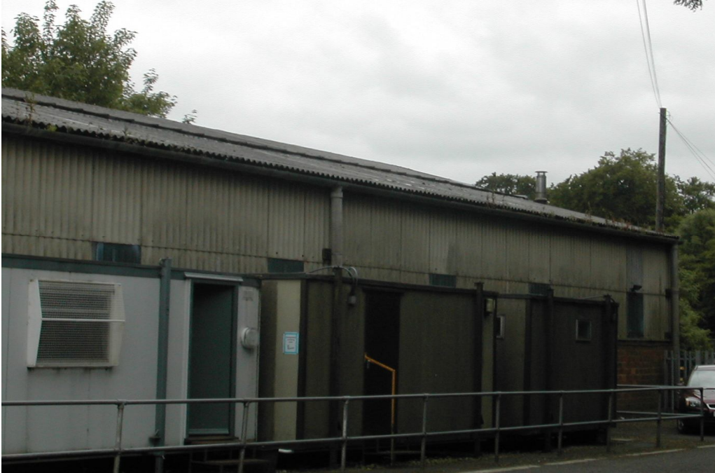
'Temporary' welfare facilities adjacent to building
