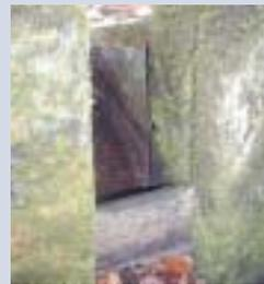
This stone hatch shows the grooves for the insertion of sluice boards. Grass kept under control to prevent the structure becoming overgrown and hidden from view.
