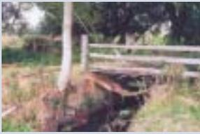
This tree is causing damage to an otherwise quite sound brick sluice structure. Roots are growing into the
