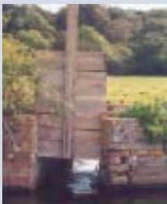
The small brick hatch is at the point where unless repairs are carried out soon there is danger of extensive collapse. Rebuilding using salvaged materials is required, though only the top five
