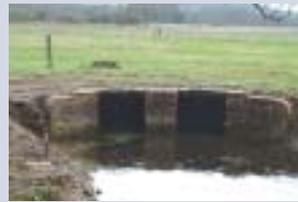
Rebuilt structure using salvaged bricks and new metal sluice boards.
