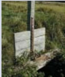
Smaller sluice board with original metal fixing mechanism. Boards raised and lowered manually without mechanised assistance.
