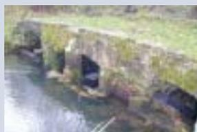
This three arch sluice structure has been carefully repointed with lime mortar and vegetation
