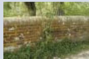
This vegetation should be carefully removed. If allowed to grow, its root system could cause significant damage to the brick parapet.
