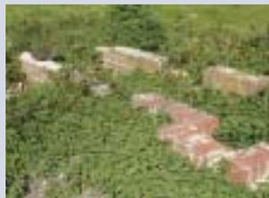
Brick aqueduct which has become overgrown. Careful cutting back of vegetation required and
