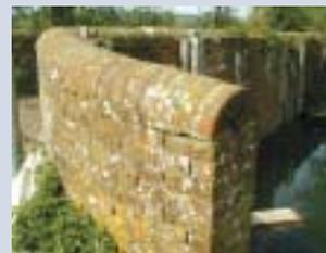
This brick constructed bridge/sluice is in generally good condition, requiring only localised repointing in lime mortar where joints are deeply eroded.
