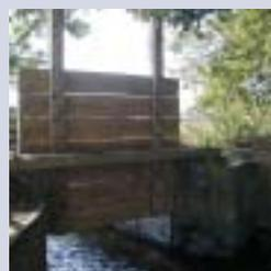
New sluice boards in position. Some brick repair required to sides of channel at lower levels.
