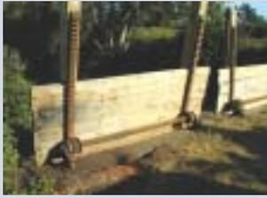
Salvaged timber and ironwork used in conjunction with new timber. Existing brickwork repaired and reinstated.
