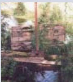
This sluice structure on the River Avon has deteriorated badly. Further delay of the horizontal timber support will result in loss of the cast iron lifting mechanism into the water.
