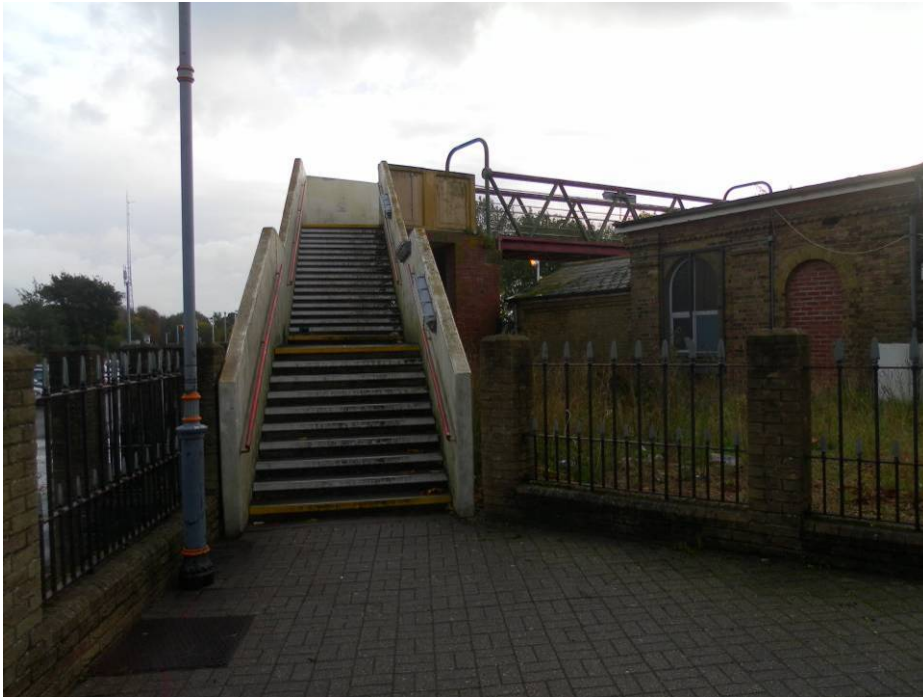
Photo 4.5 - Steps up to the footbridge over the railway from the north side
