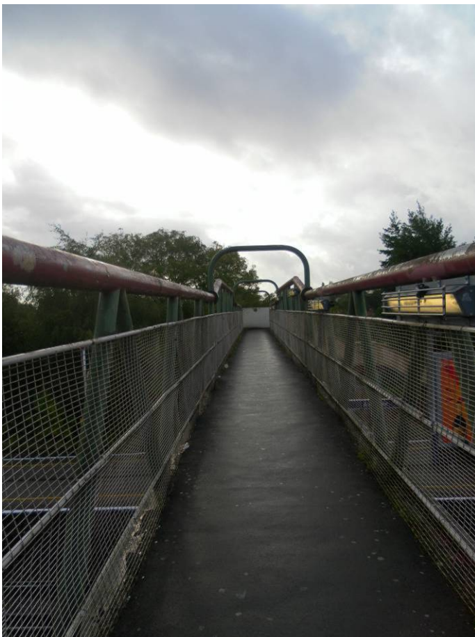
Photo 4.6 - Footbridge over the railway
