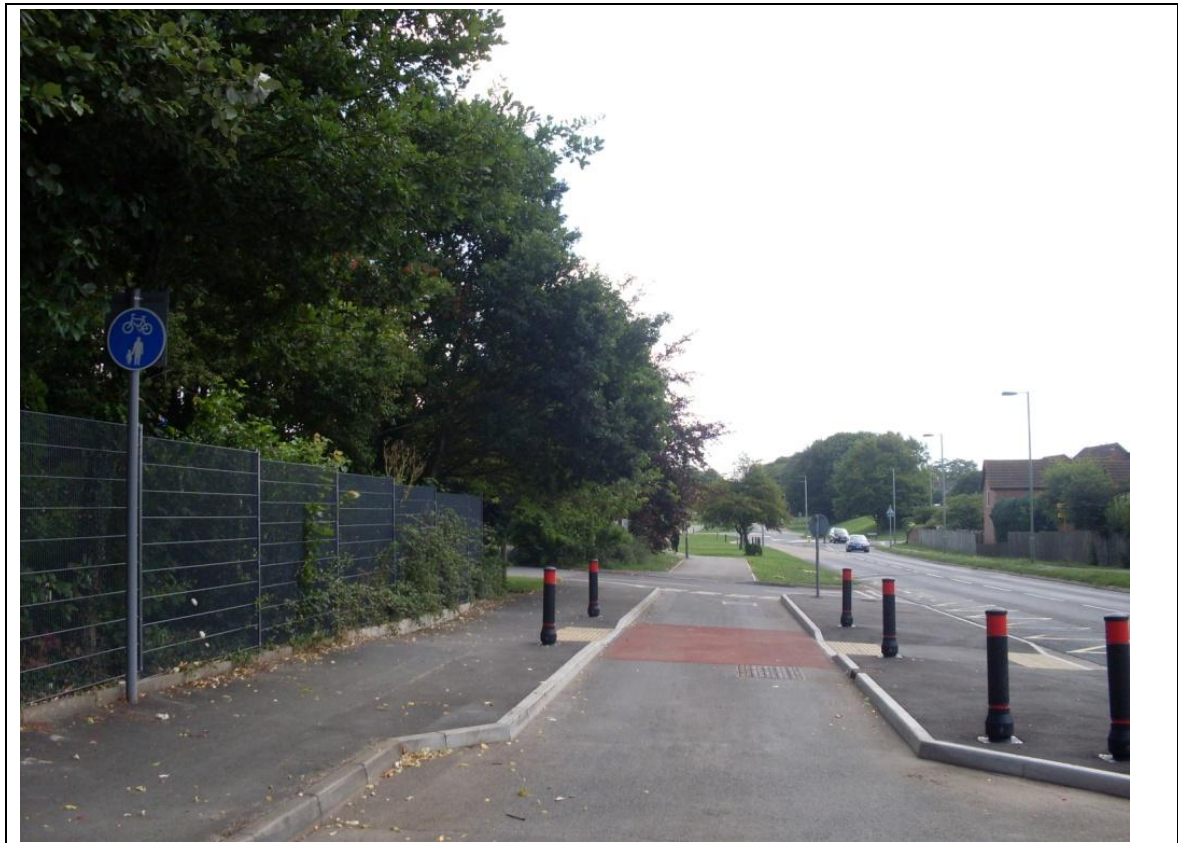
Figure 3.5 Photo of Pedestrian and Cycle Facility on Smannell Road
