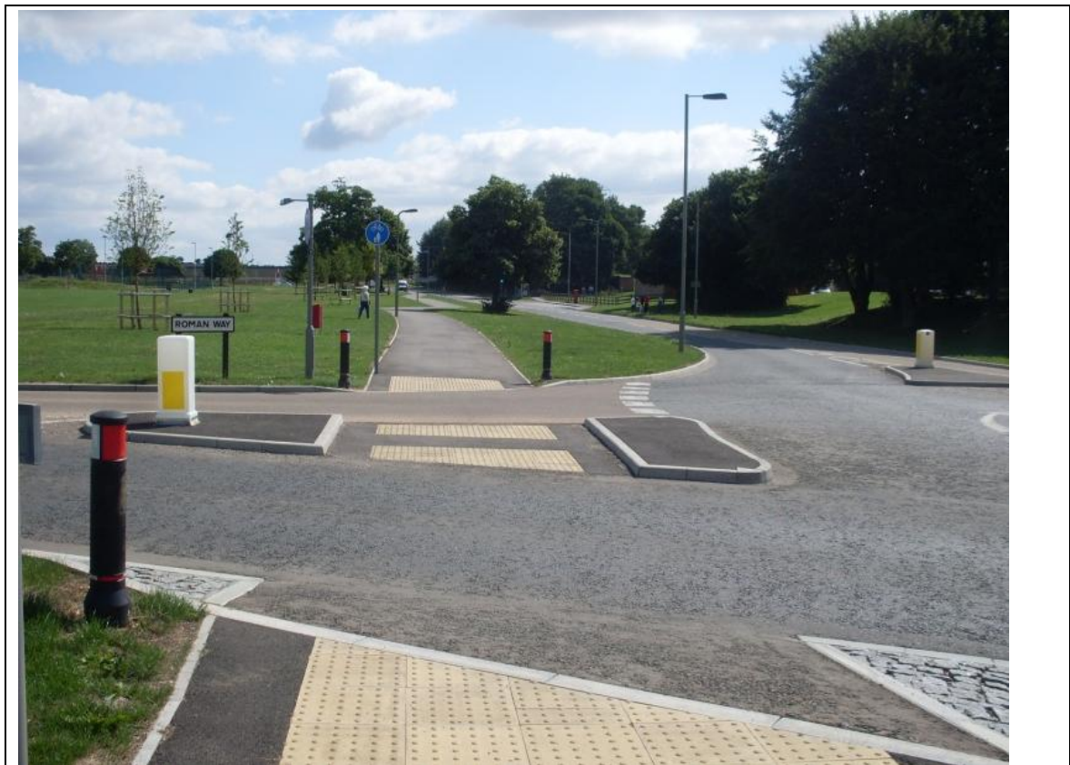
Figure 3.6 Photo of Pedestrian and Cycle Facility on Smannell Road
